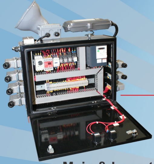
Main & Long travel Control Panel
